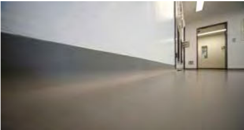
Floor-Wall Connection with Sikafloor® and SikaGard® WallCoat.
